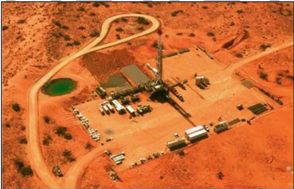
Plate 3-12: Petroleum exploration drilling showing typical layout of well lease (Source: Santos 2003)
