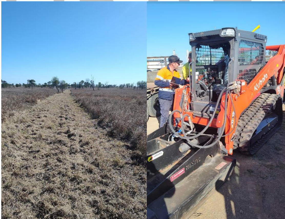
Plate 3-9: Prepared seismic line following use of Bobcat mounted vegetation mulcher in tall / dense pasture grass (Source: M.Kneipp, 2026)
