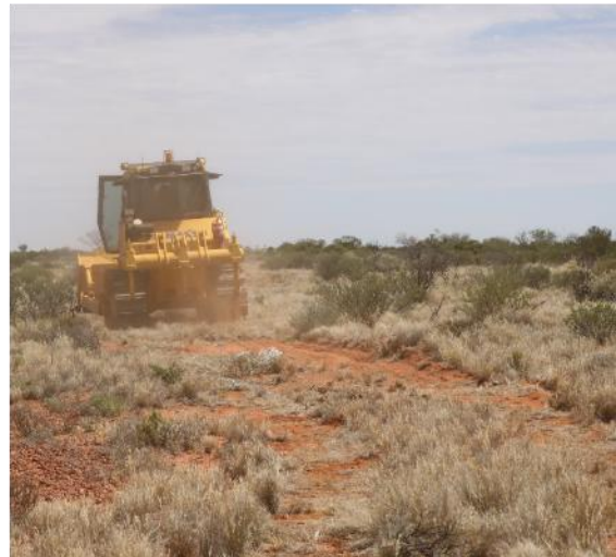
Plate 3-10: Preparing a seismic line using a grader and dozer, with the blade just skimming the surface to remove hazards but leaving rootstock (Source: M.Kneipp, 2026)
