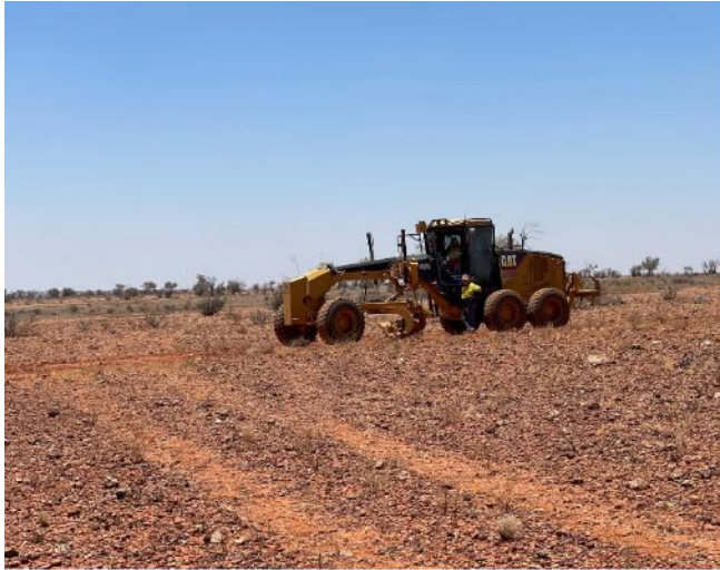
Plate 3-10: Preparing a seismic line using a grader and dozer, with the blade just skimming the surface to remove hazards but leaving rootstock (Source: M.Kneipp, 2026)
